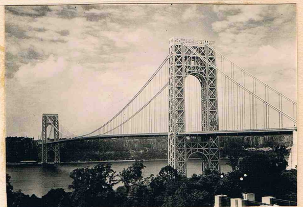
George Washington Bridge
